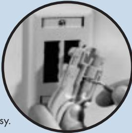
**2.** Push color-coded conductor pairs into the 110 termination until they stop, leaving a maximum .5" of cable unjacketed. The correct wiring configuration for both 568A and 568B is clearly indicated on the jack module.
