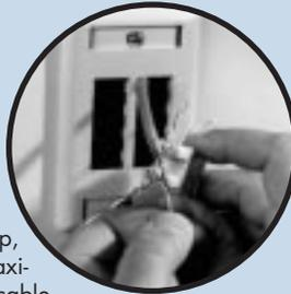
**3.** Place the P&S punchdown tool against a pair and press. The tool automatically seats and trims each conductor — while creating reliable, high-performance connections. Repeat for each pair, then place the included gray stuffer caps onto the 110 terminations.
